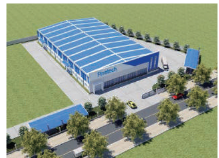
New factory under construction in Vietnam
