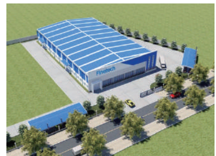
New factory under construction in Vietnam
